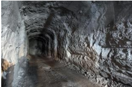
Demonstration tunnel 420 m
