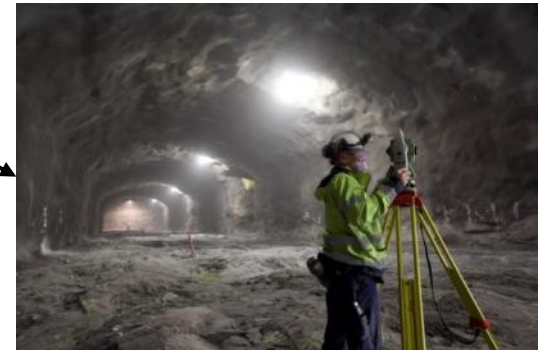
Technical tunnels 455 m
