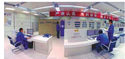
Fig. 5 – The hot test of the CNNC 404 Pilot Plant [4]
